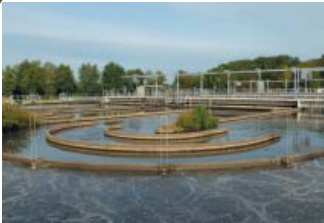
Waste Water Treatment
